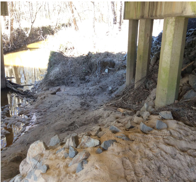
PHOTO 1 Description Erosion at bent 6
