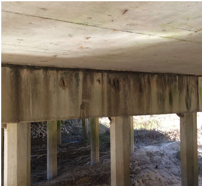
PHOTO 1 Description Rebar exposed bent 5 cap east face
